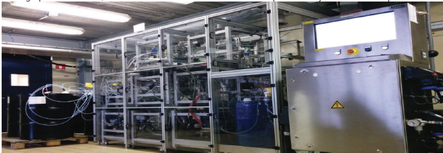
Pilot Continuous Flow Installation
